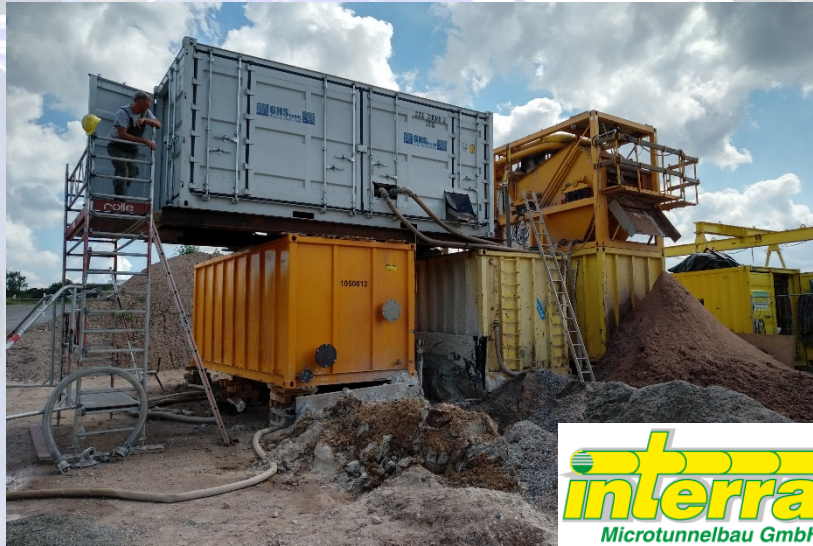
➤ GHT 390_ Baustelle Furth/ Erlangen 2017 (interra)
